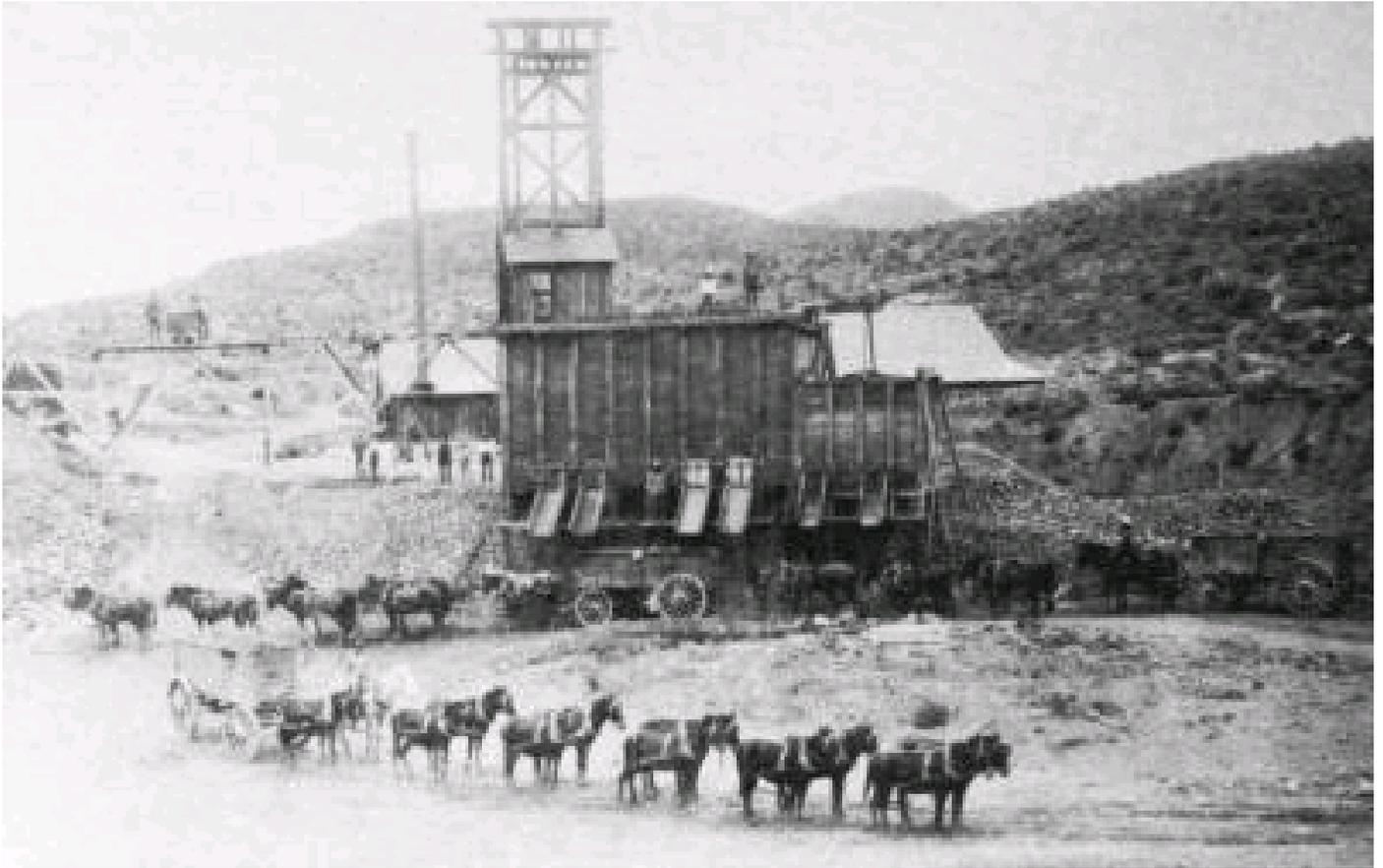
**The Shafter Silver Mine-**The processed silver ore was hauled in sacks by wagon trains under guard to Marfa, Texas to be transported by rail to an El Paso, Texas smelter for refining to 99.9% purity level as “fine silver” for the commercial market. The photograph was drawn from the work of David Brooks
